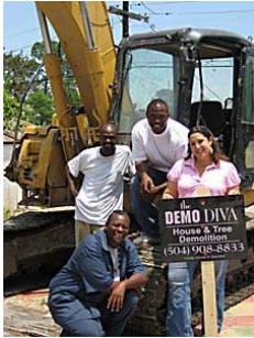
Demo Diva Simone Bruni and her crew work hard to give local homeowners a clean slate for rebuilding.
